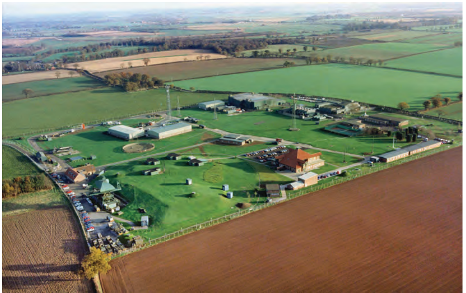
RAF Neatishead from the air. The R3A bunker is bottom left with the Type 84 radar to its left. The R12 (Type 85 radar) building is top right with the WWII happidrome (now the Defence Radar Museum) to its right. In the centre the radio masts and the adjacent buildings will all be retained by the MoD when the site is sold.
